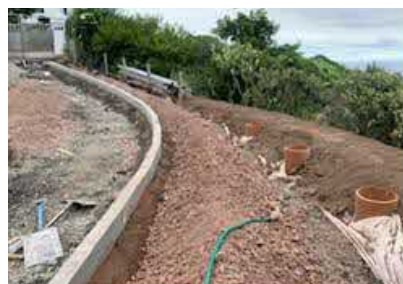
New kerbing installed and preparation for the new path
