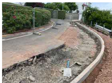
Road being prepared for re tarmacing
